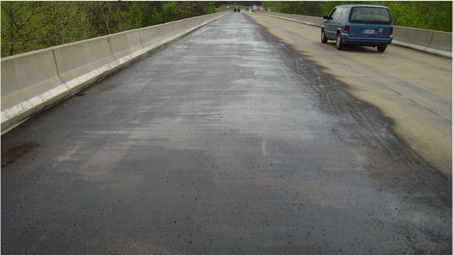
Typical bridge deck seal
